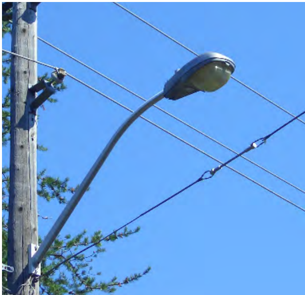
Figure 3.12 Example of Existing Cobra Light Fixture Photo by R. Johns
